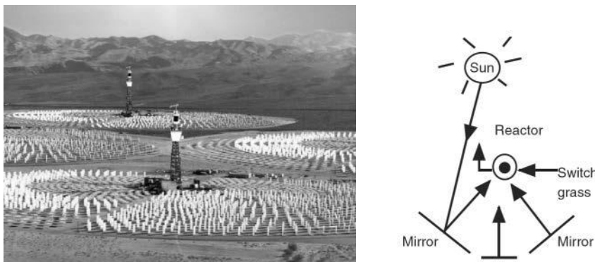
Figure P8-16.1 Solar field design. Five 265-m-tall towers with three heliostat fields/tower, on 275 acres of land in Daggett, CA. Net concentration 3,868 suns and 295 MW delivered to each solar reactor. (Melinda M. Channel, Jonathan Scheffe, Allan Lewandowski, and Alan W. Weimer, November 11, 2009. Also see: Chemical Engineering , 116, p. 18, March 2009).
