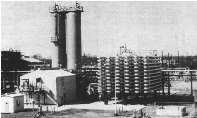
Figure 2-9 Dimersol G (an organometallic catalyst) unit (two CSTRs and one tubular reactor in series) to dimerize propylene into olefins. Institut Français du Pétrole process. Photo courtesy of Editions Technip (Institut Français du Pétrole).
